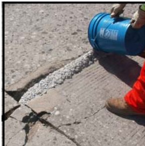
Pour into the spall which can be filled to grade as the material is free flowing and self leveling.
