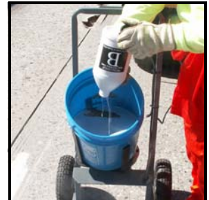
After shaking the contents of bottle "B" for 20 seconds, pour the contents into the 5 gallon pail.
