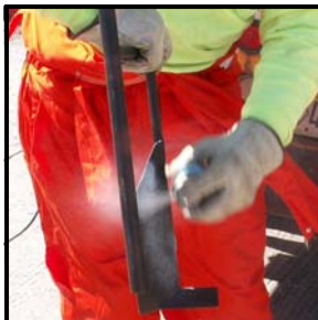
Spray a light coat of vegetable oil on the paddle. Acting as a release agent, it will keep the paddle clean.
