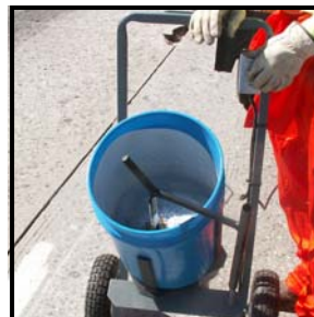
Place the paddle in the pail, turn on the switch and mix for 1 minute. You are now ready to add aggregate.
