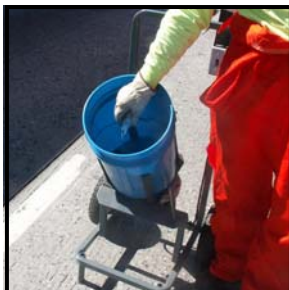
On cold days or where a very quick cure is required, supplied catalyst may be added to speed the reaction.
