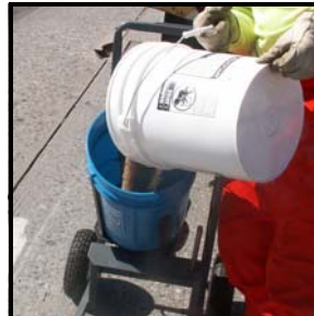
Pour the supplied 30 pounds of specially coated aggregate into the pail, covering the A side.
